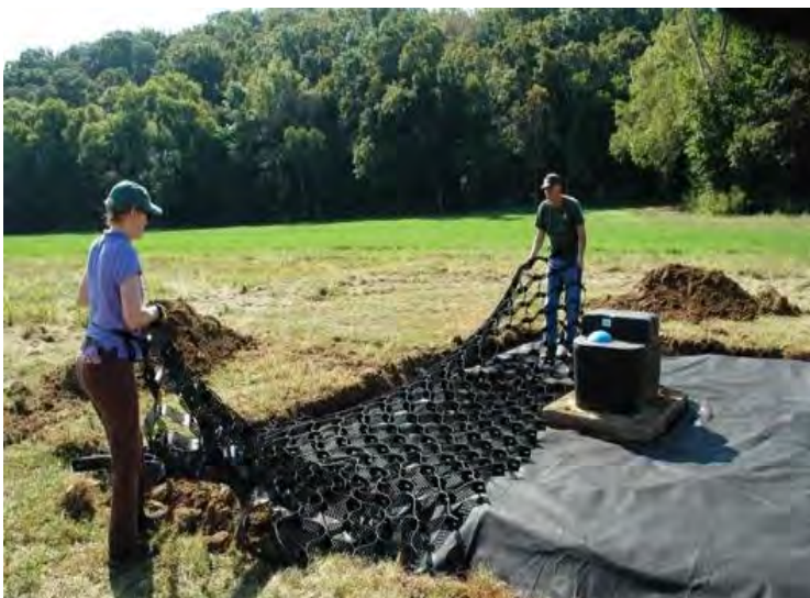
Installing a stabilized alternative livestock watering system in SCWW.
